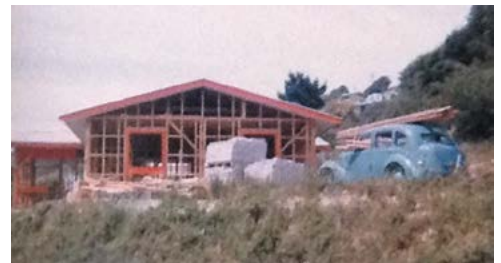
Building our first home. Note the red lead primer used on Windows and fascia board!!
