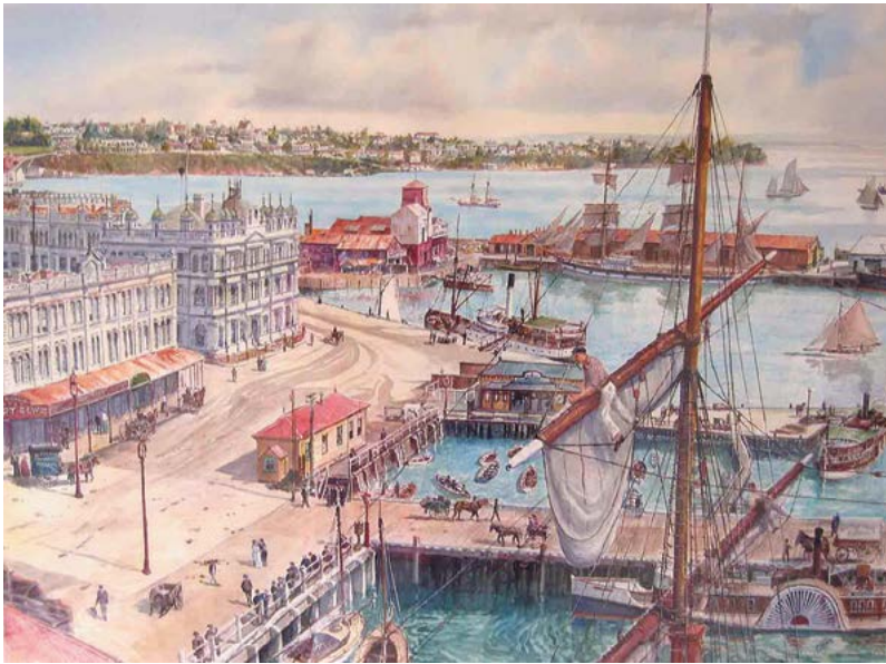
View of old Auckland from the level of the masthead of a ship looking south-west over Queen's Wharf towards St. Mary's Bay and Ponsonby, circa 1904. Watercolour. 730 x 530mm.
