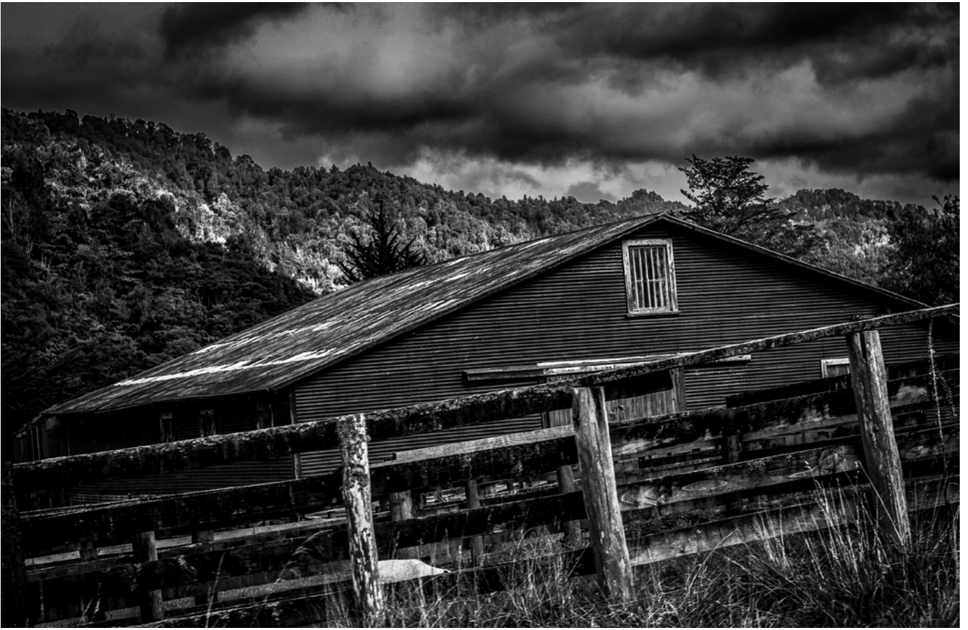
4288 x 2848 35mm Digital Photograph. A farm shed for shearing and stock
